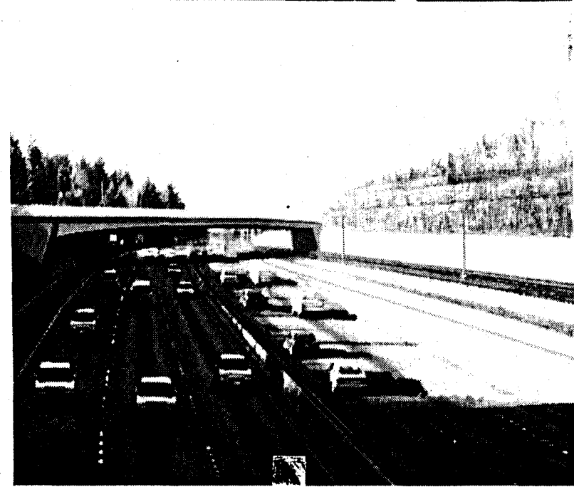
VIEW FROM CAMELOT CT. OVERPASS LOOKING WEST NORTHSIDE AND SOUTHSIDE OPTIONS
